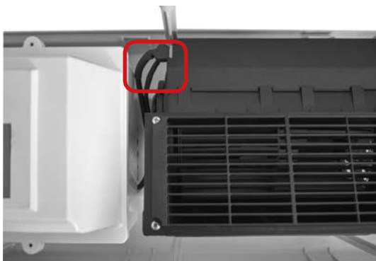
Fig. 7.4.2.6: Connecting the fan plug
